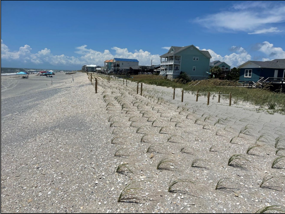
Figure 2-23: Recently planted section of dune (M&N photo 7/25/22)
