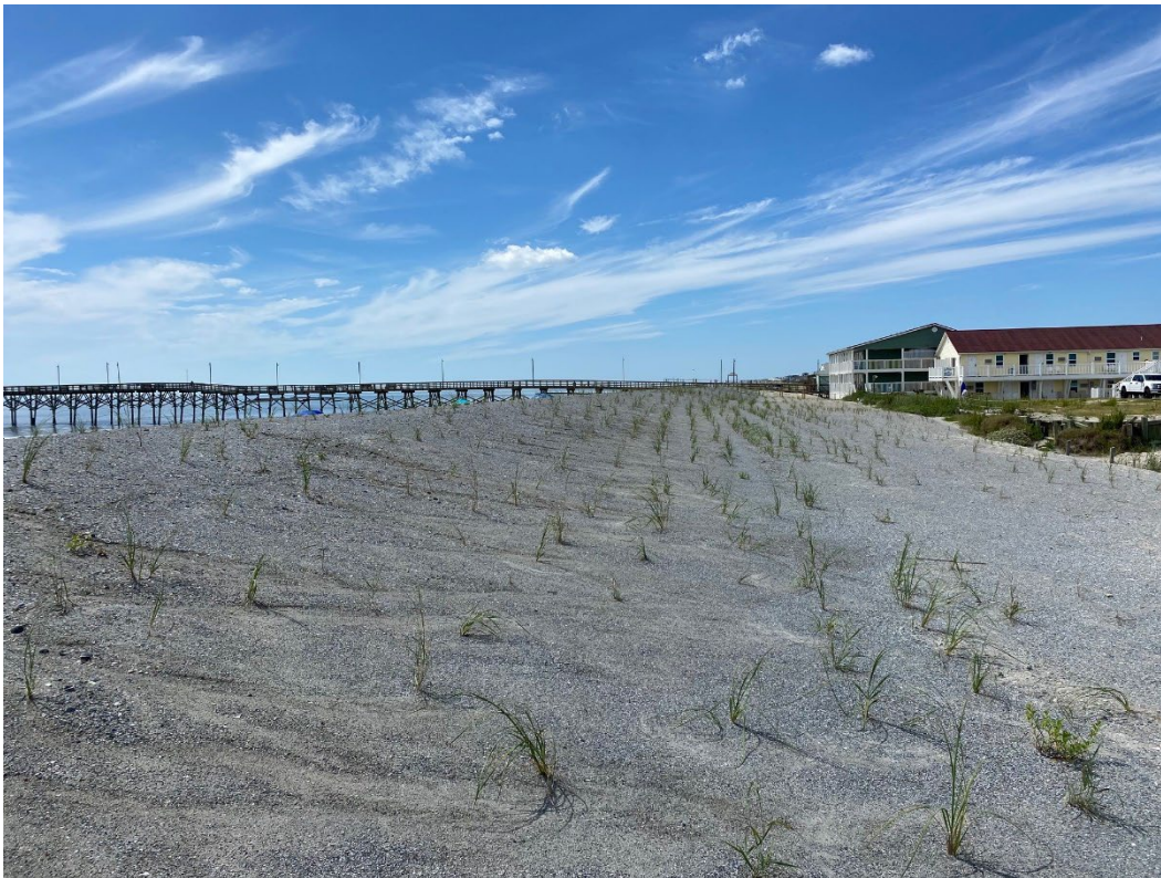
Figure 2-14: Recently planted section of dune (M&N photo 6/15/21)
